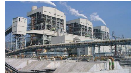
TNB Manjung 4 Coal-Fired Power Plant, Malaysia
