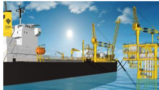
Ikdam FPSO, Bertam oil field in PM307, off Peninsular Malaysia
