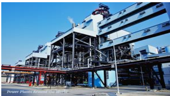
Tuas Power Station Combined Cycle Power Plant 5 (CCP5), Singapore
