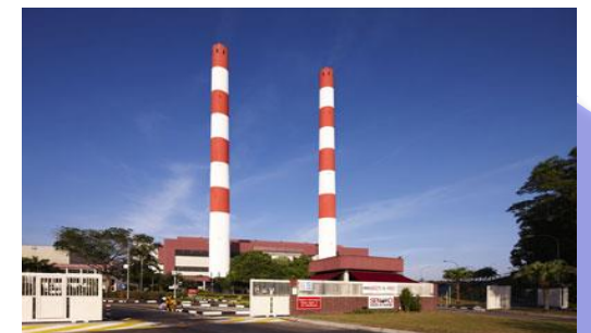
TuasOne Waste-to-Energy Plant, Singapore
