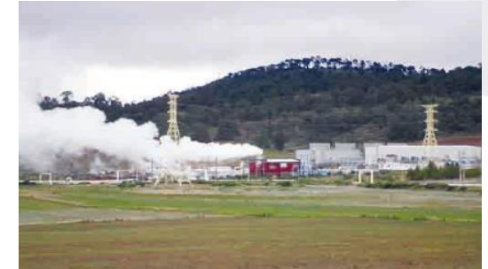
Domo De San Pedro Geothermal Power Plant, Mexico
